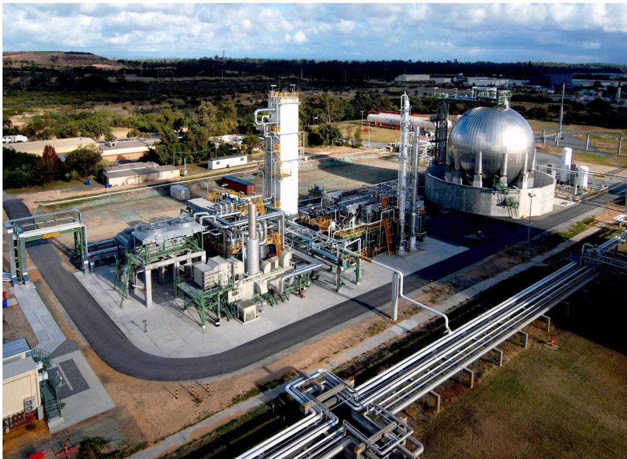
Figure 16 LNG Plant, Kwinana, Australia. 61ktpa with Spherical Storage. Source: Linde Engineering.
