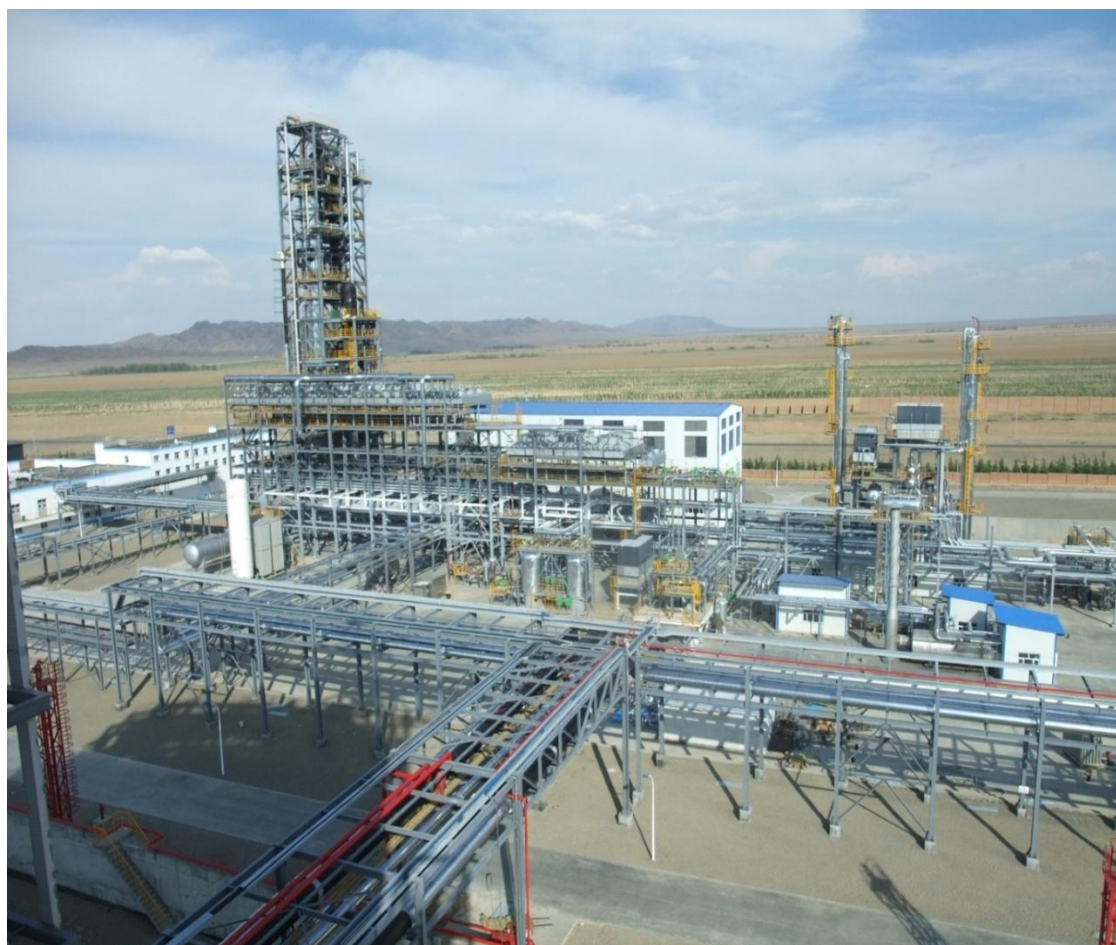
Figure 13 The 440ktpa LNG plant at Guanghui, China. LIMUM® - CWHE Process with integrated N2-Removal. Source: Linde Engineering.
